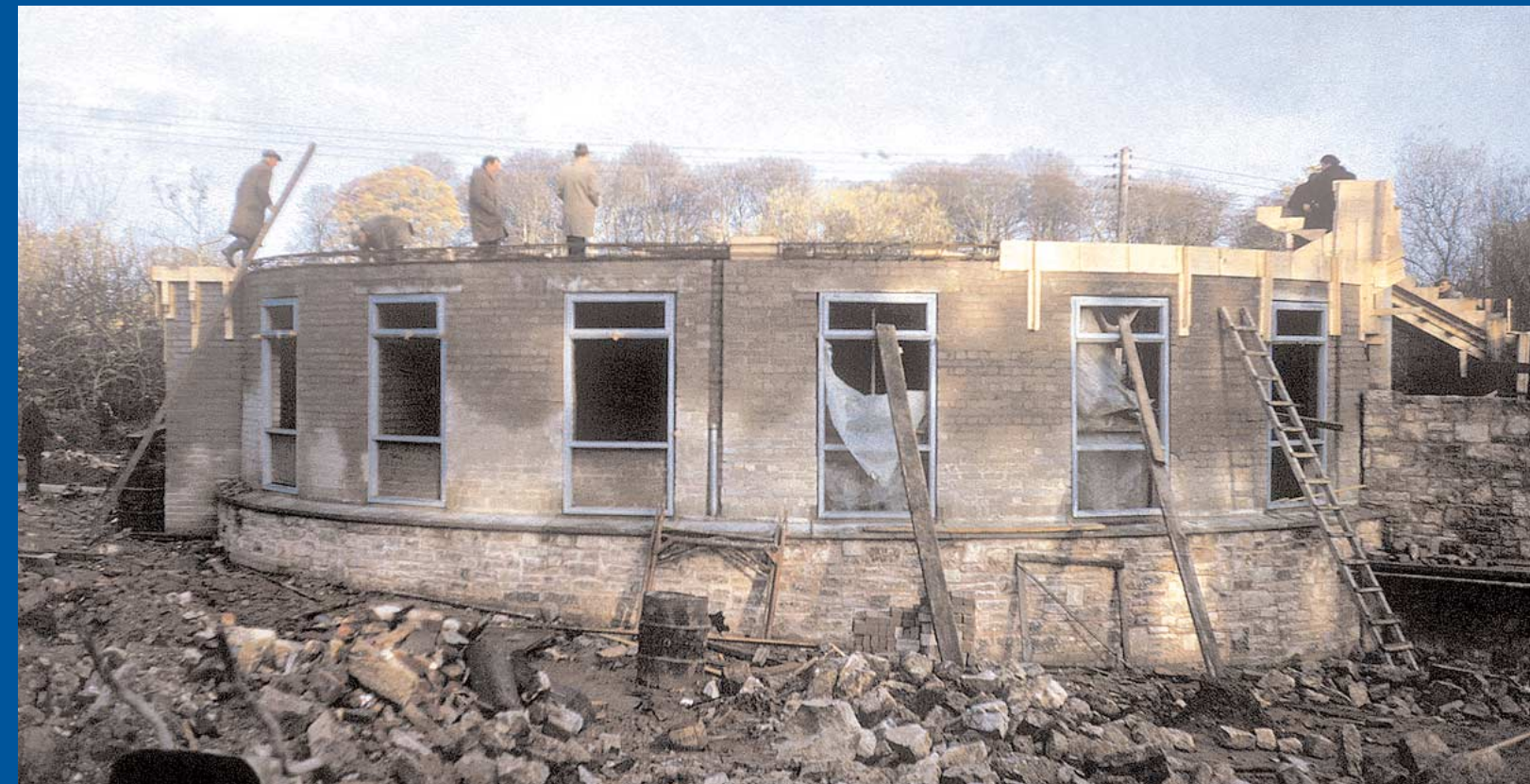
The first floor completed: 1966
