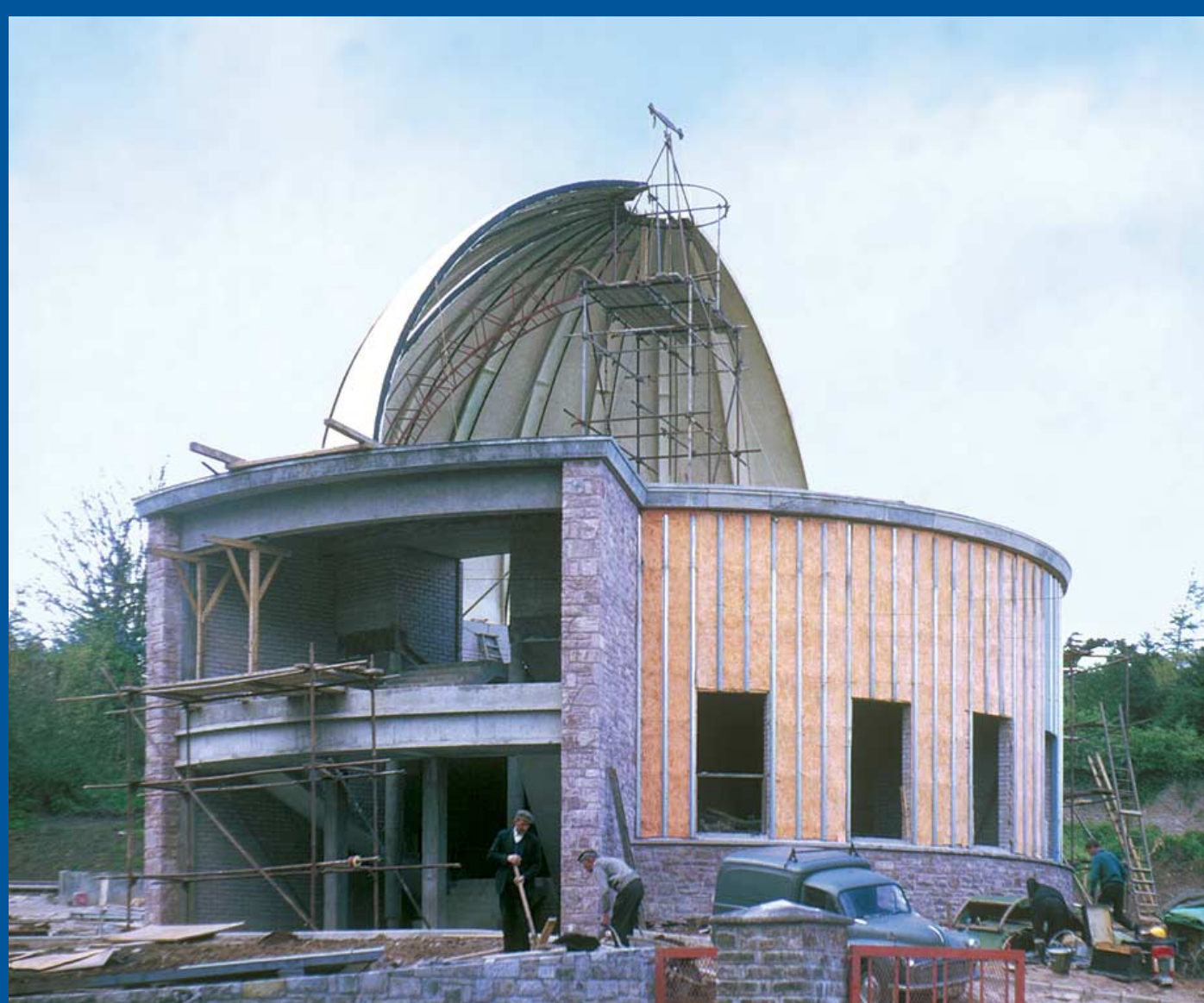
The dome takes shape: 1967
